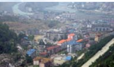
Overview of building damage at Beichuan County town.
