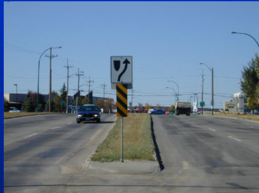
Airport Drive Median
